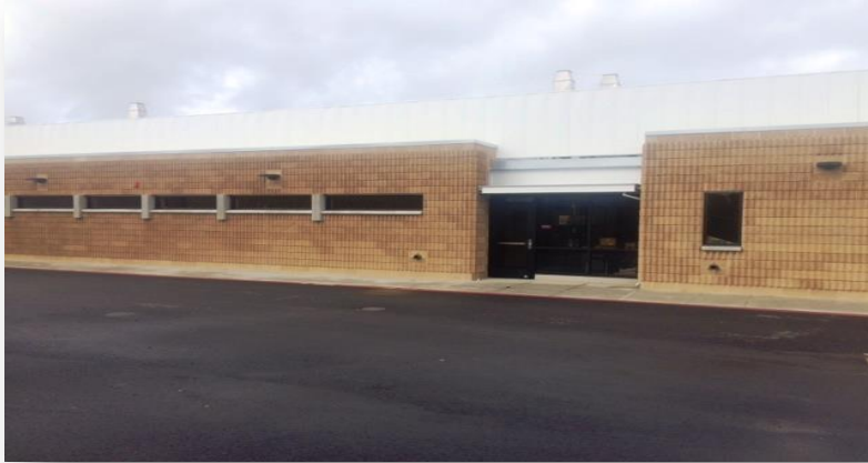
TPHS – J Bldg. Chemistry Classrooms
