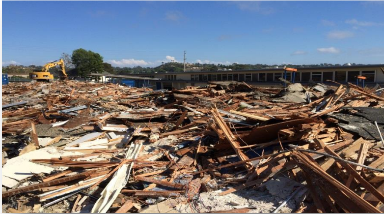
EWMS – Campus Re-construction
