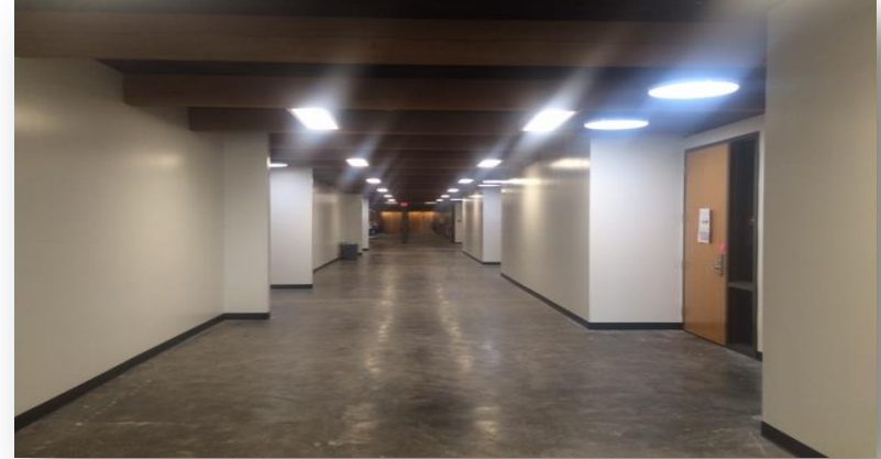
TPHS – B Bldg./HVAC
