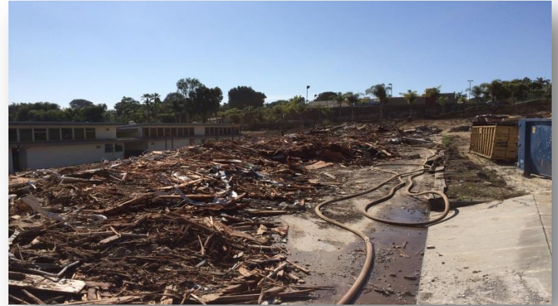
EWMS – Campus Re-construction
